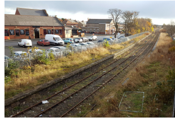
Newcastle - Northumberland Rail Line - £94.2m
